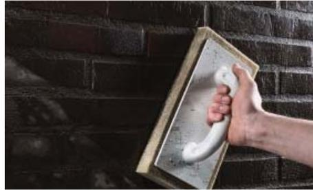
The excess grout is washed off diagonally using a plaster float with a sponge or foam pad
