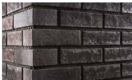
The finished joint pattern, which will be flexible and efflorescence free. Full masonry stretches are grouted at one go.
