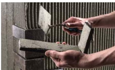
The corner angles are worked using the floating-buttering method
