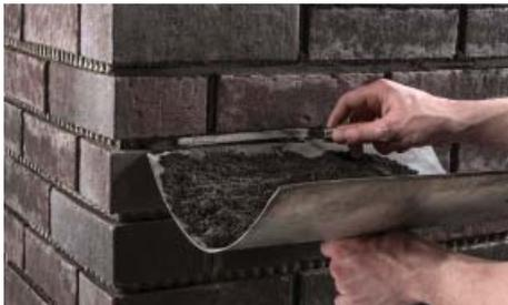
Conventional grouting using a pointed trowel and metal float along the horizontal
