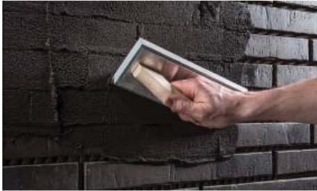
With the slurry method, the joints are filled diagonally with the grouting or plaster float. Walls should be worked from top to bottom
