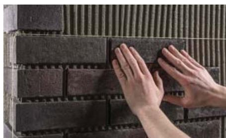
Use a string line to plumb the brick area. The brick slips are pressed into the adhesive bed
